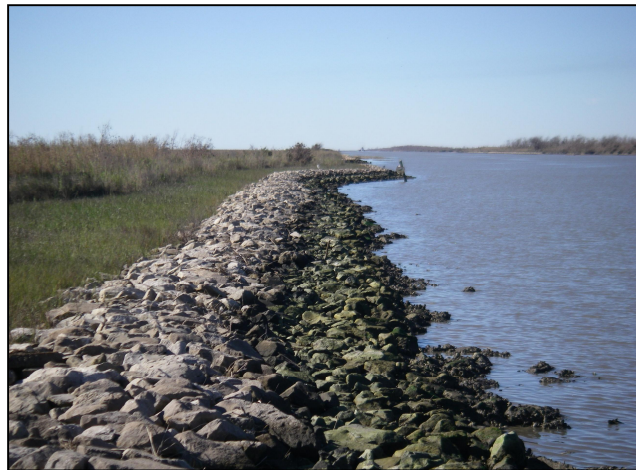
Figure 4. Typical Breakwater structure along GIWW
