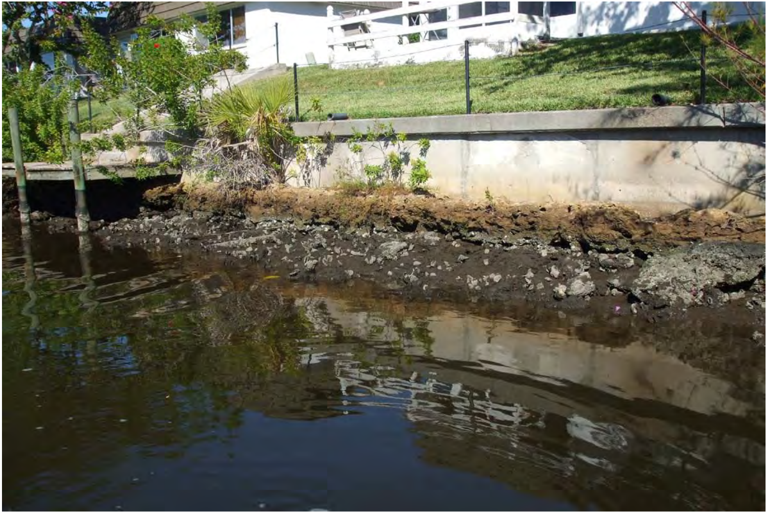
SCATTERED CLUMPS – SC AND SCATTERED SHELL - SS Clumps and shells are scattered in the mud along the base of the seawall
