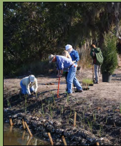
Volunteers working together to plant native vegetation in zones just above the oyster shell bags.
