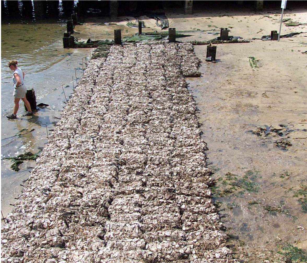
Figure 5.1. Bags filled oyster shells along the shoreline to form reefs. SC Aquarium SCORE reef building project, Charleston SC. Photo courtesy of Loren Cohen, Shellfish Research Section, Marine Resources Research Institute, South Carolina Department of Natural Resources, Charleston, SC.
