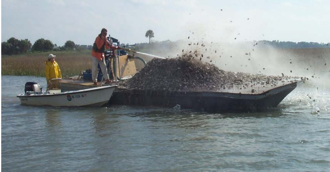
Figure 4.1. Large-scale reef restoration shell planting in 2002, Folly Creek, Charleston Co., South Carolina, Andy Jennings running the water pressure nozzle. Photo courtesy of Loren Cohen, Shellfish Research Section, Marine Resources Research Institute, South Carolina Department of Natural Resources, Charleston, South Carolina.
