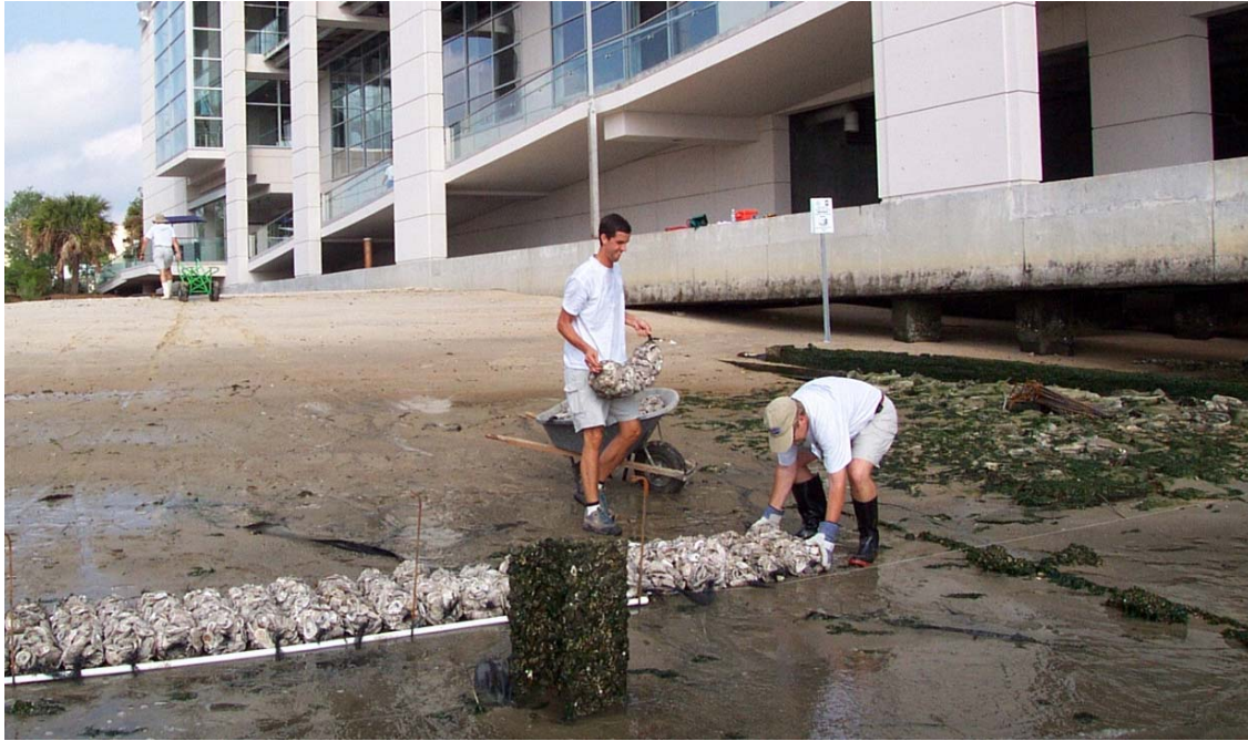
Figure 5.0. South Carolina Aquarium SCORE reef building project, Charleston SC reef bags Individuals placing bags filled with oyster shells along the shoreline. Photo courtesy of Loren Cohen, Shellfish Research Section, Marine Resources Research Institute, South Carolina Department of Natural Resources, Charleston, SC.
