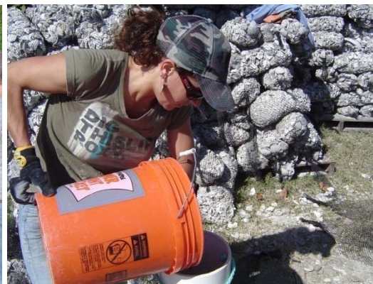
Filling shell bags with fossil shell and deploying these to construct oyster reefs in Clam Bayou. Photo credits: SCCF staff
