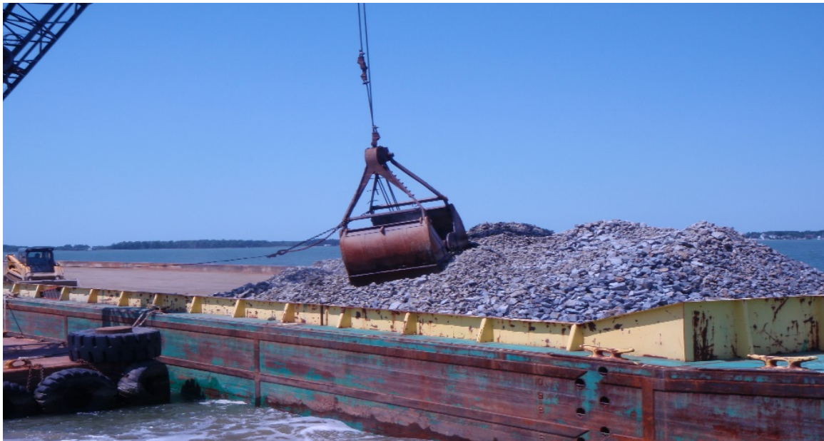
U.S. Army Corps of Engineers places rock mixture on restoration reefs in Harris Creek, Maryland. Photo: U.S. Army Corps of Engineers
