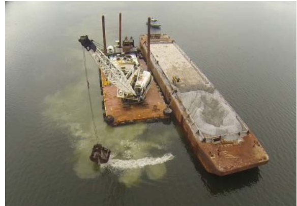
Dredged shell being placed on Great Wicomico River. Photo: U.S. Army Corps of Engineers
